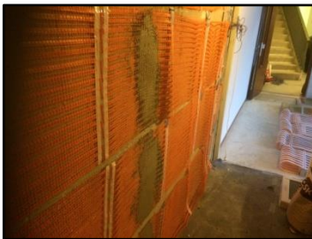
Wall and floor heating in a renovation project
