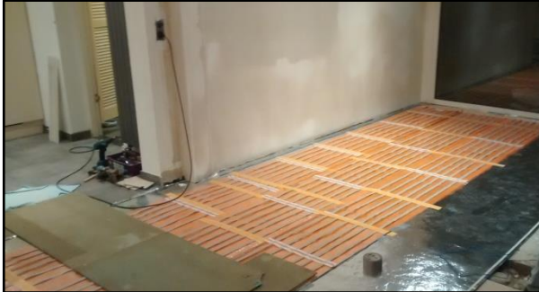
Floor heating in a new build home, applied under non glued laminate
