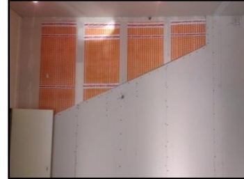
(Prefab) wall heating
