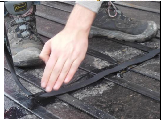
Fixing the heating cables
