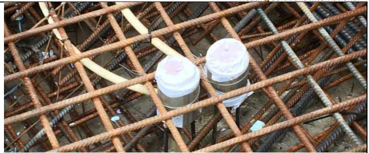
Preparation of temperature and moisture sensor.
