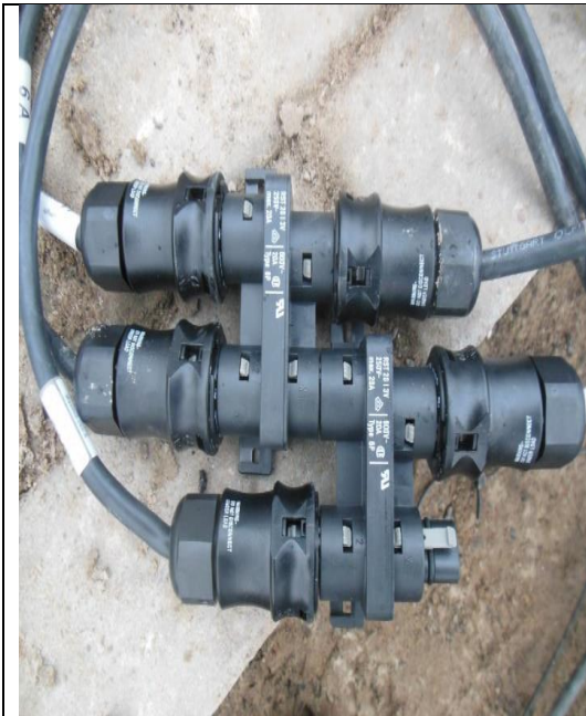
Junction boxes: Wieland connectors IP 68.
