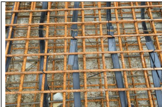
Heating ribbons fixed on Iron
