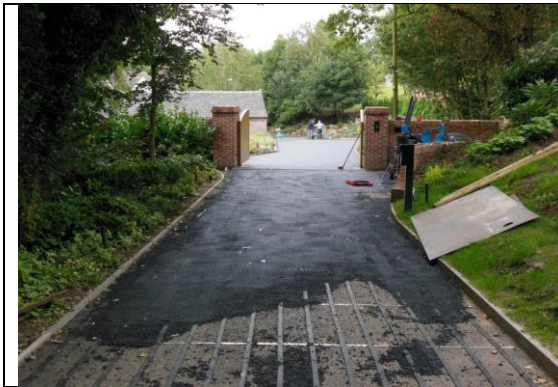
Heating ribbons fixed first layer and below first asphalt layer.
