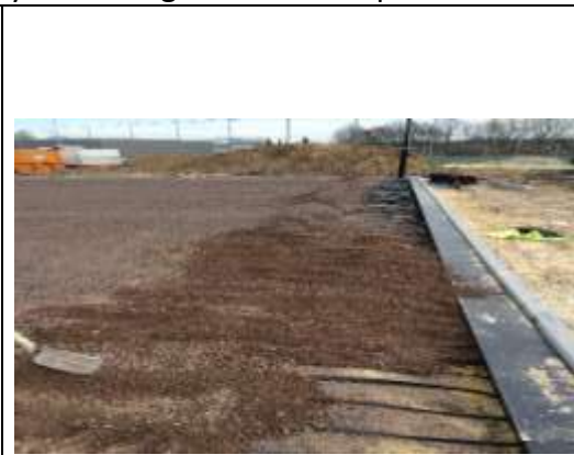
Installation of a cable gutter with entry of heating ribbons on top side
