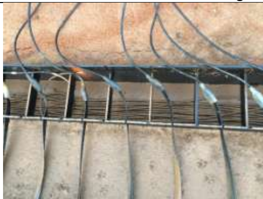
Installation of a cable gutter with entry of heating ribbons on top side
