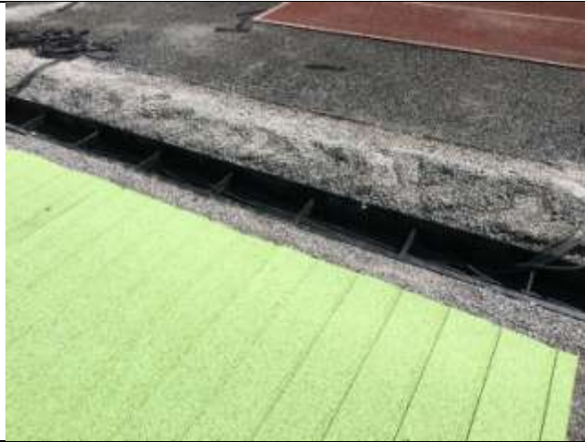
Installation of a cable gutter with entry of heating ribbons on top side
